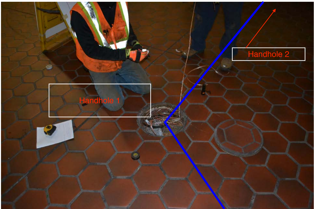
Photo #2 – E02 Shaw-Howard U South: Handhole 1 to Handhole 2
