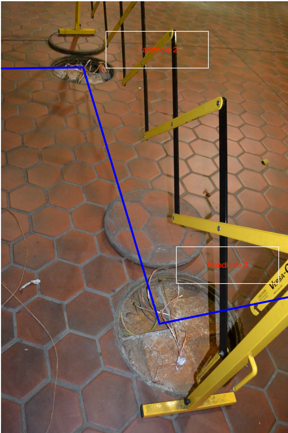
Photo #3 – E02 Shaw-Howard U South: Handhole 2 to Handhole 3
